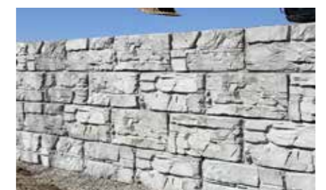
MaxumStone Retaining Wall
