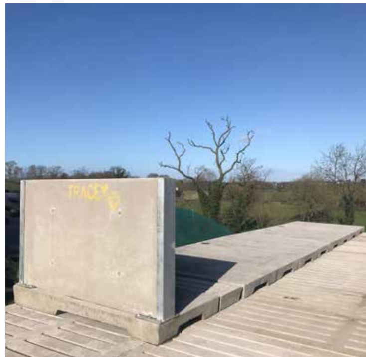
Cubicle end wall
