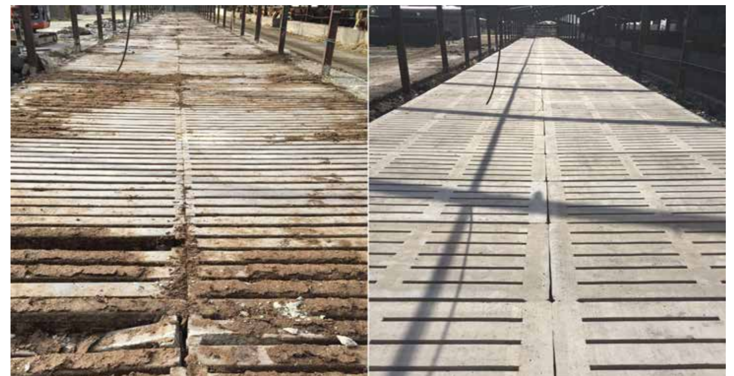
Refit before & after
