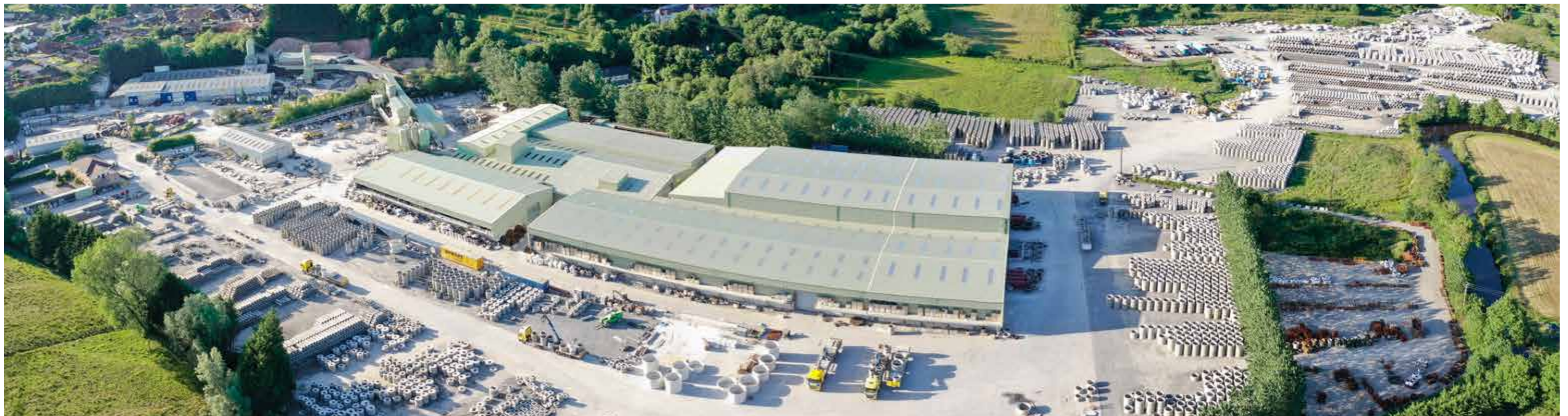
Tracey Concrete's Precast Drainage Factory - Enniskillen
