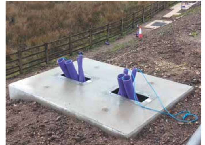
Precast communication installed
