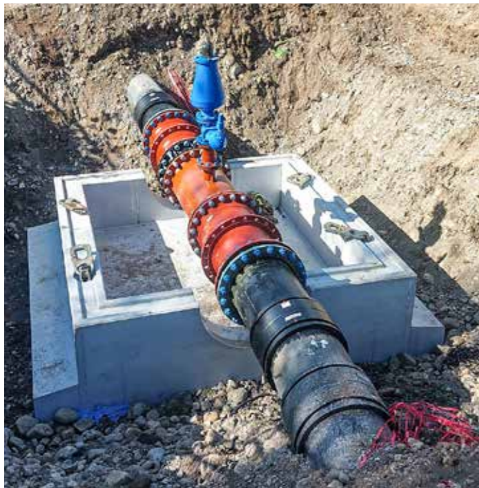
Tongue & groove joint prior to riser installation
