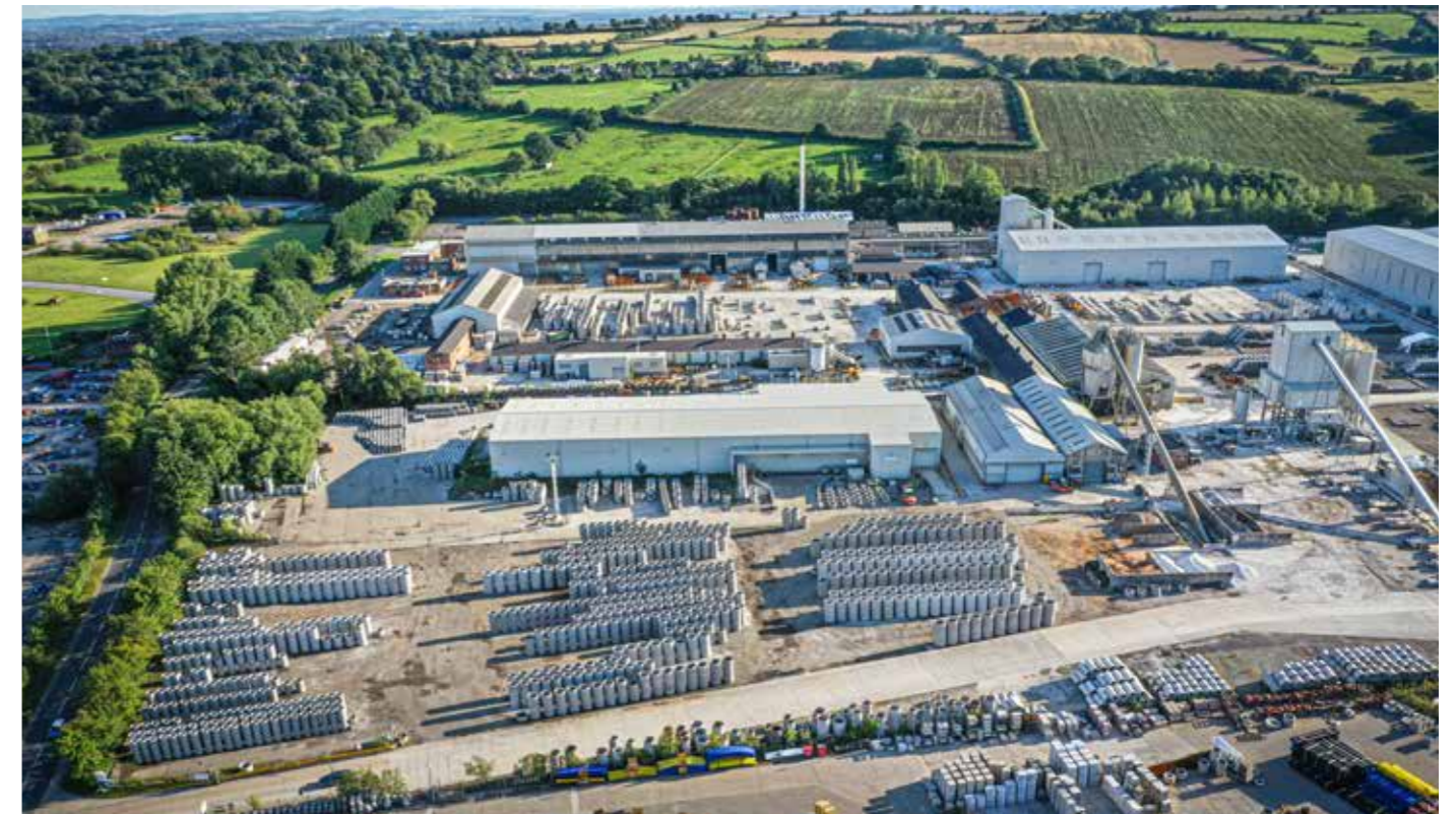
Tracey Concrete's Precast Factory - Stanton
