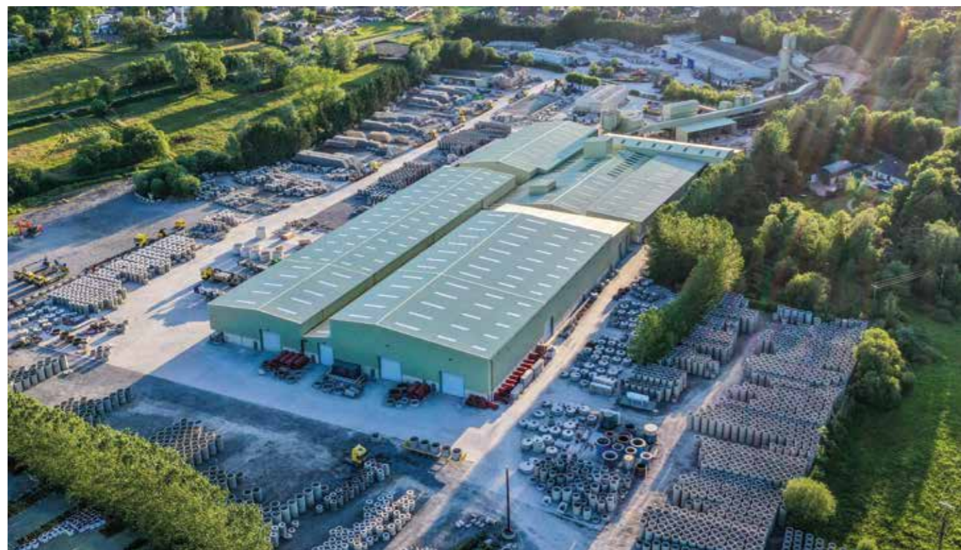
Tracey Concrete's Precast Factory - Enniskillen
