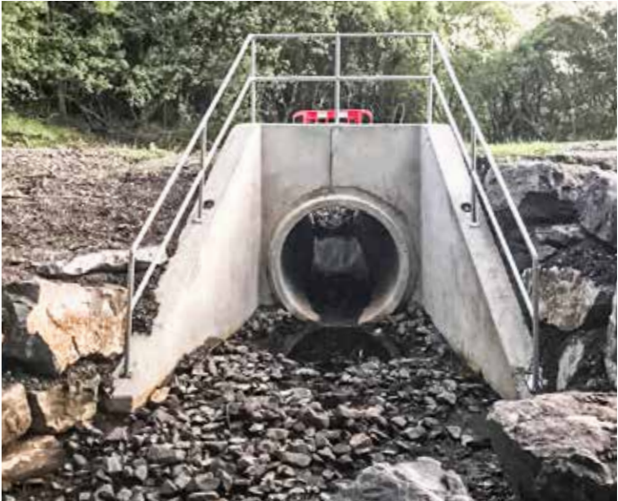
Steps & handrails & extended toe piece
