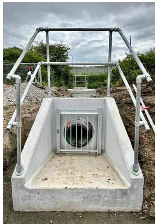
Small Headwall, hand railings & grate installed
