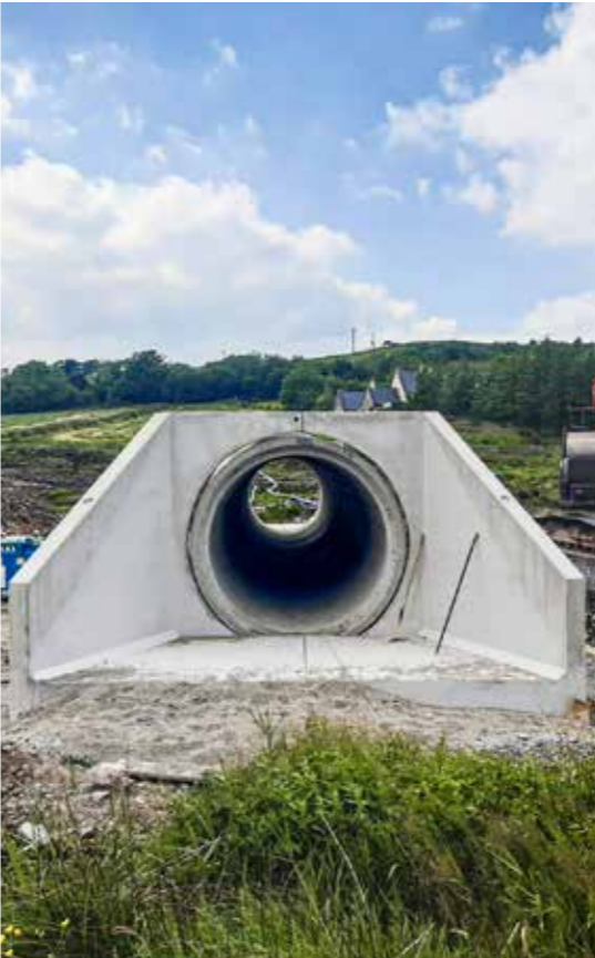
XXL Headwall install completed
