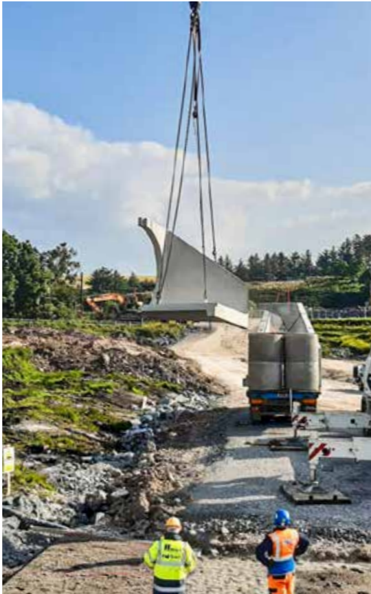
XXL Headwall lift during install
