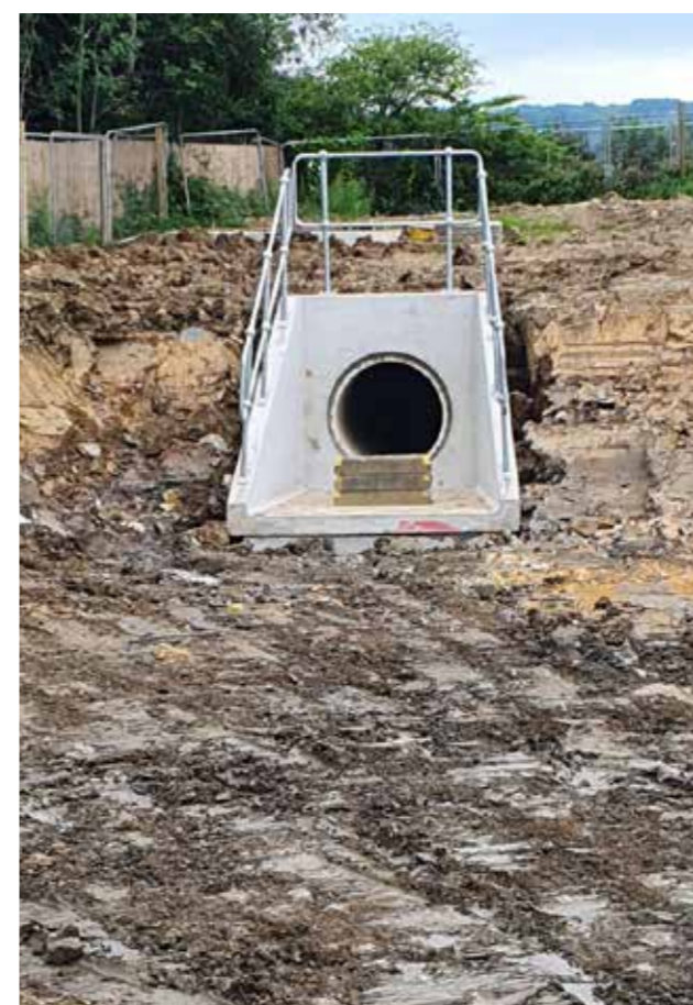
Medium Headwall installed with hand railings fitted
