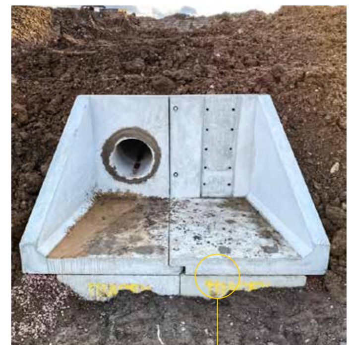
Installed Toe Piece
