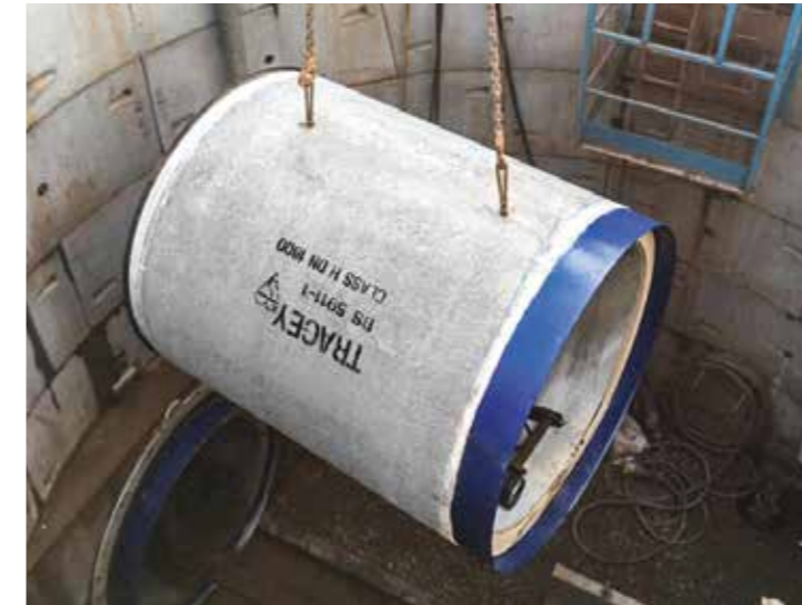
Precast jacking pipes being lowered into launch shaft
