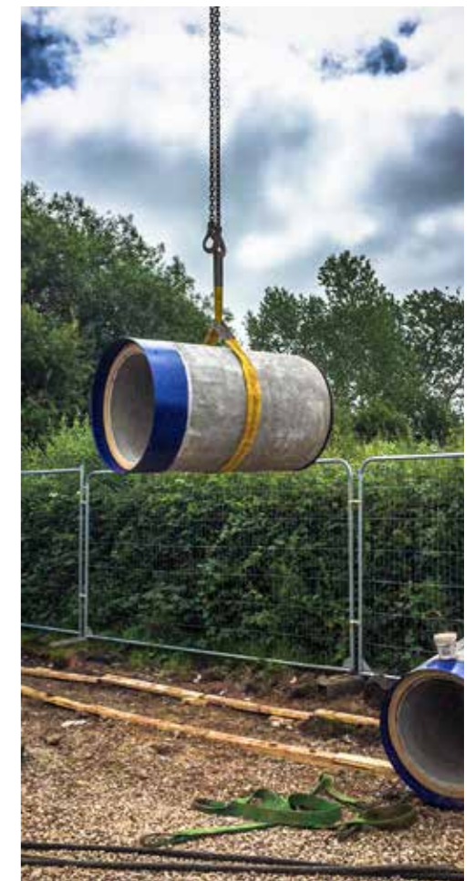
Standard jacking pipe lifted with sling and chain onsite during installation
