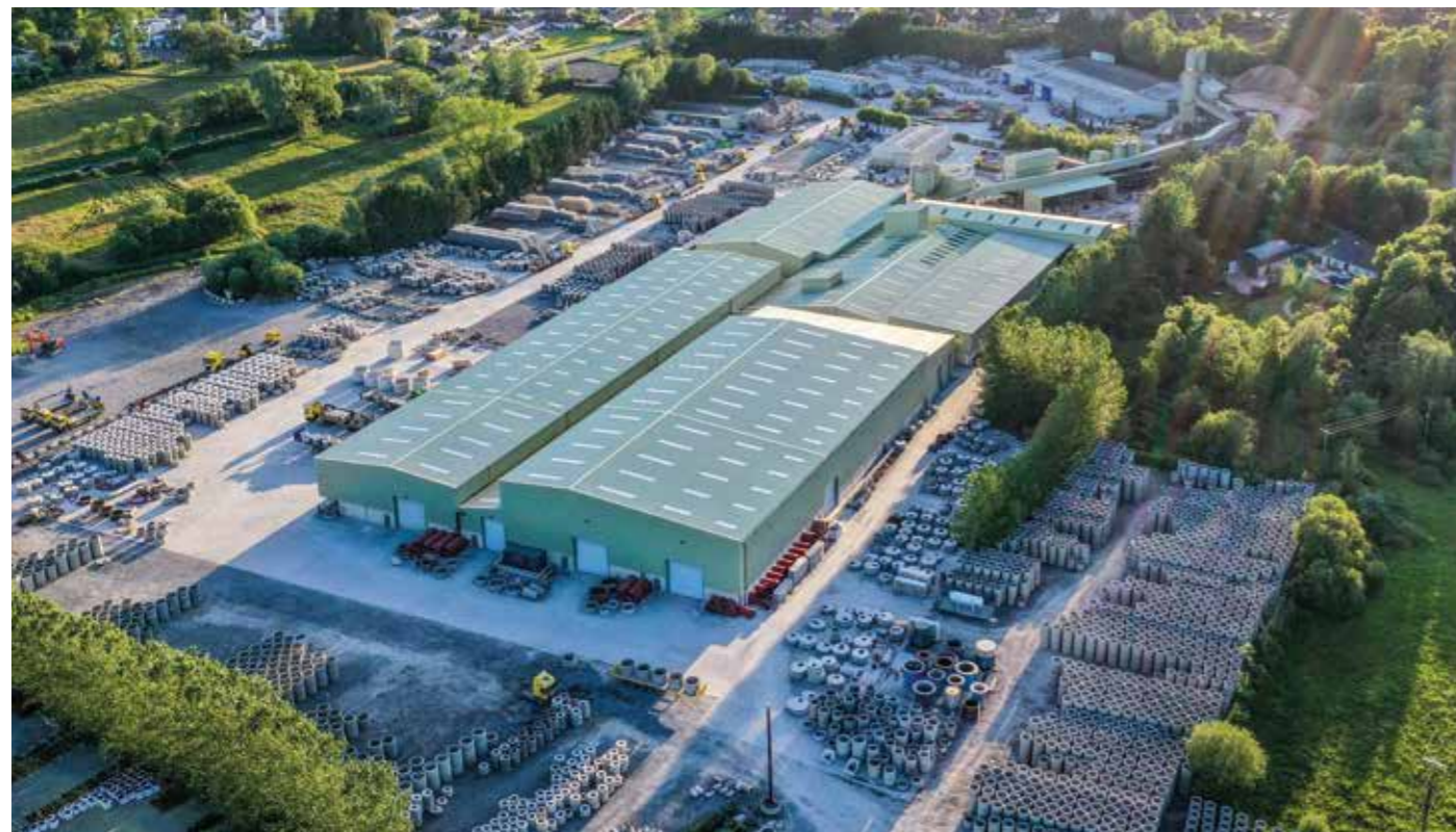
Tracey Concrete's Precast Factory - Enniskillen
