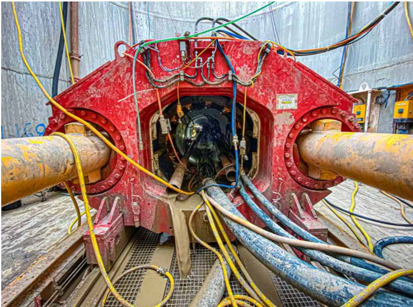
Jacking pipe frame
